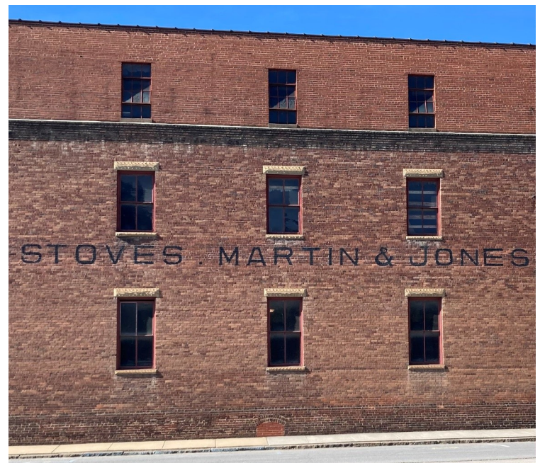
Figure 3. Exterior of 422 West Edgar Avenue, 2021.
